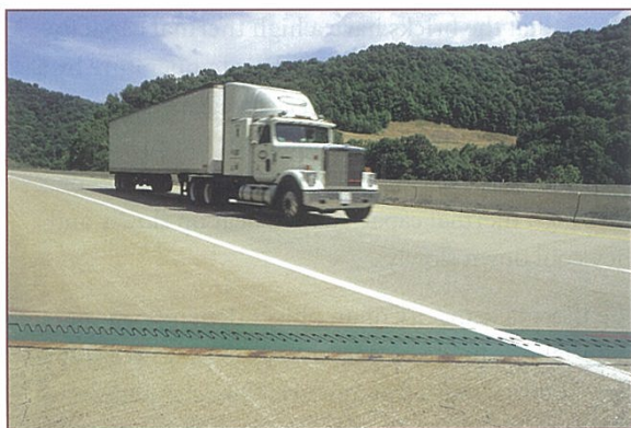
Figure 10.12 This truck is about to cross an expansion joint on a motorway bridge. On a hot day, the bridge expands and the interlocking 'teeth' of the joint move closer together.
