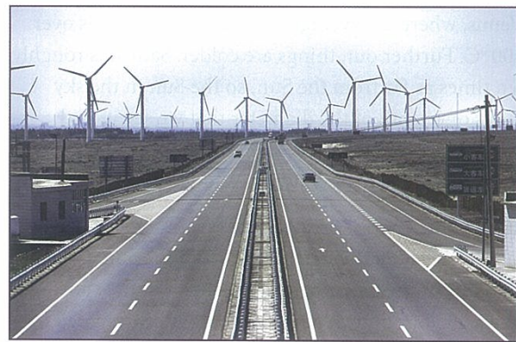
Figure 7.4 These giant turbines are part of a wind farm at Xinjiang in China. They produce as much electricity as a medium-sized coal-fired power station.
